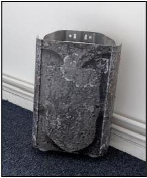
Close up view of the antenna wrapped in a vinyl image of the section of the castellation parapet where the antenna will be
